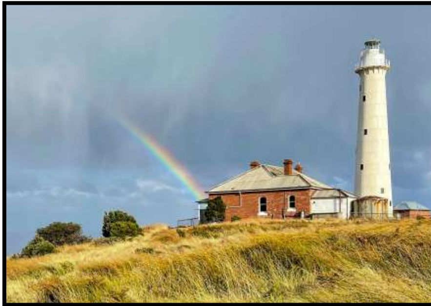
There's a pot of gold on the restored front verandah of lightkeeper's quarters No 3 at Tasman Island!
