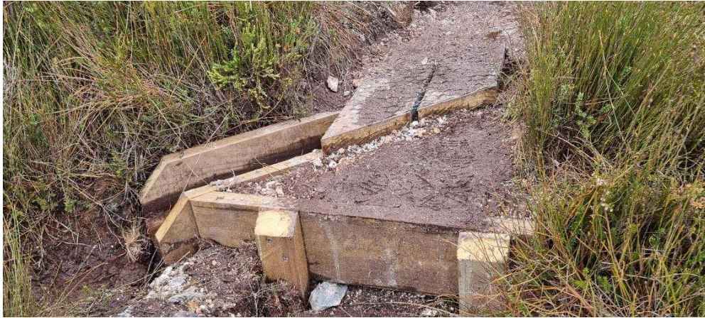
Photo by Mark Devine of a new step and gutter on Clyde's Hill track
