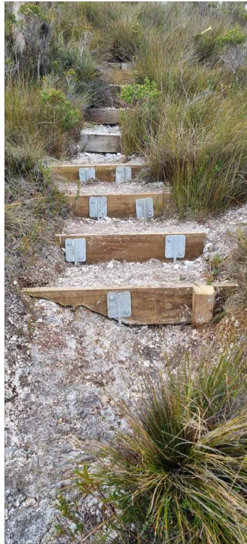
Photo by Mark Devine of new steps made on Clyde's Hill track
