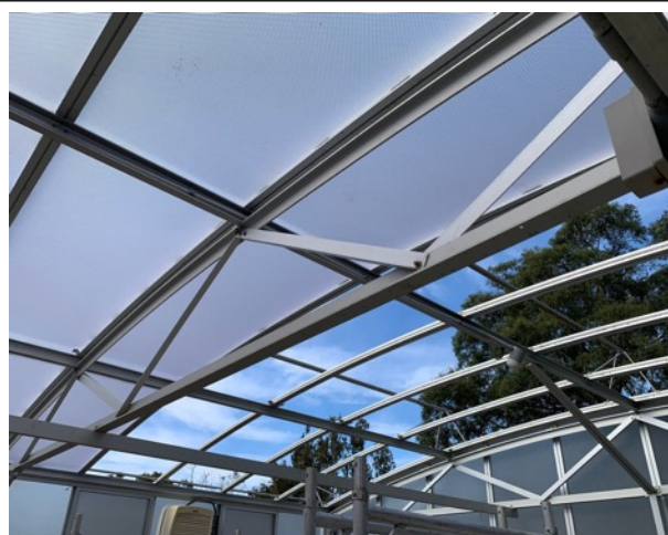
New hot house roof going up
