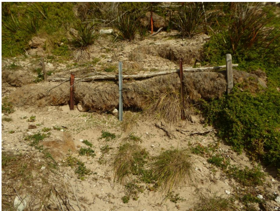
Figure 2. Current condition of erosion control structure that was installed probably about November 2012 on the East Cove slope. Photo M Comfort November 2024.
